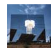
The KHI Solar One plant in Upington, South Africa. This solar thermal plant has a capacity of 50 MW, and contains around 4,000 mirrors that rotate according to the position of the sun to reflect and concentrate sunlight onto the tower. Here water is heated to evaporation and, through turbines, becomes energy.
