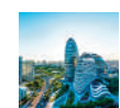
Wangjing SOHO, Beijing. The Wangjing SOHO is a multipurpose complex consisting of three towers, 115, 127 and 200 meters tall, designed as three interweaving mountains. The project was designed by Zaha Hadid Architects.
