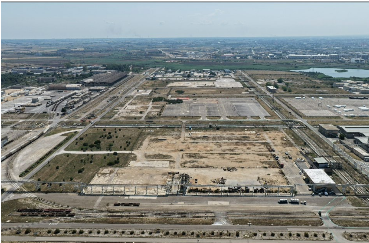
Site where the Eni Storage Systems plant will be built in Brindisi
