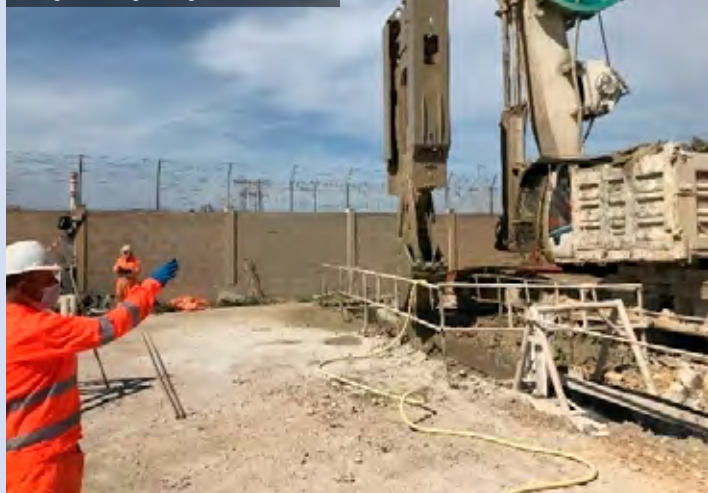
Excavation of the composite diaphragm using the Casagrande grab bucket
