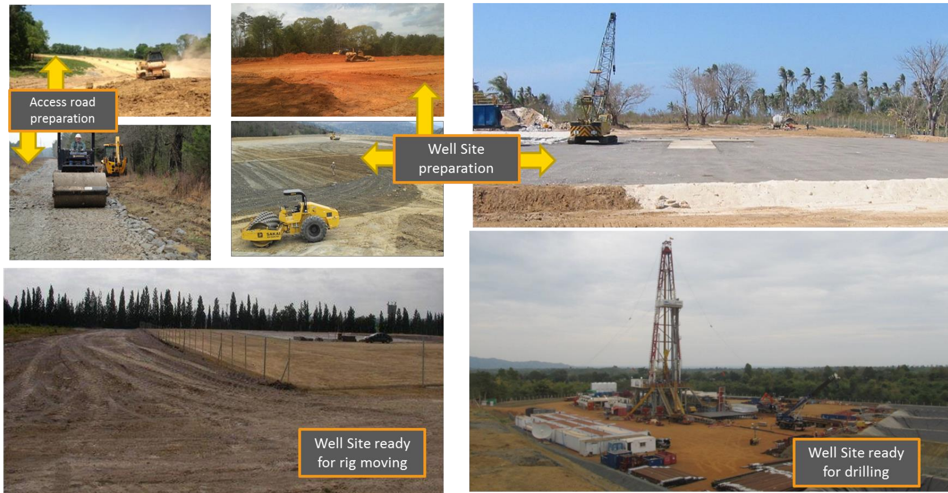
Figure 4.7: Example Images of Well Pad Construction Process
